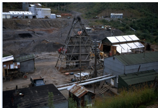
The Pre-1955 Main Processing Area, showing headworks and support buildings. The post-1955 mill is in the background.
