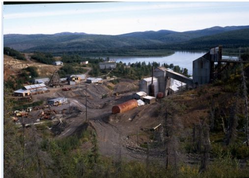
Overview of the Main Processing Area in 1969 or 1970 from the southeast.
