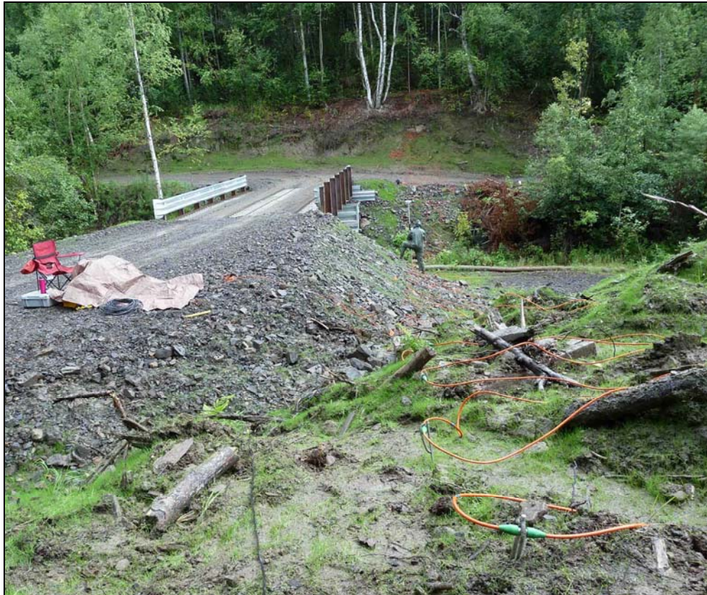
Figure 18. Photograph of the DC resistivity equipment deployed on line 6, looking northwest.
