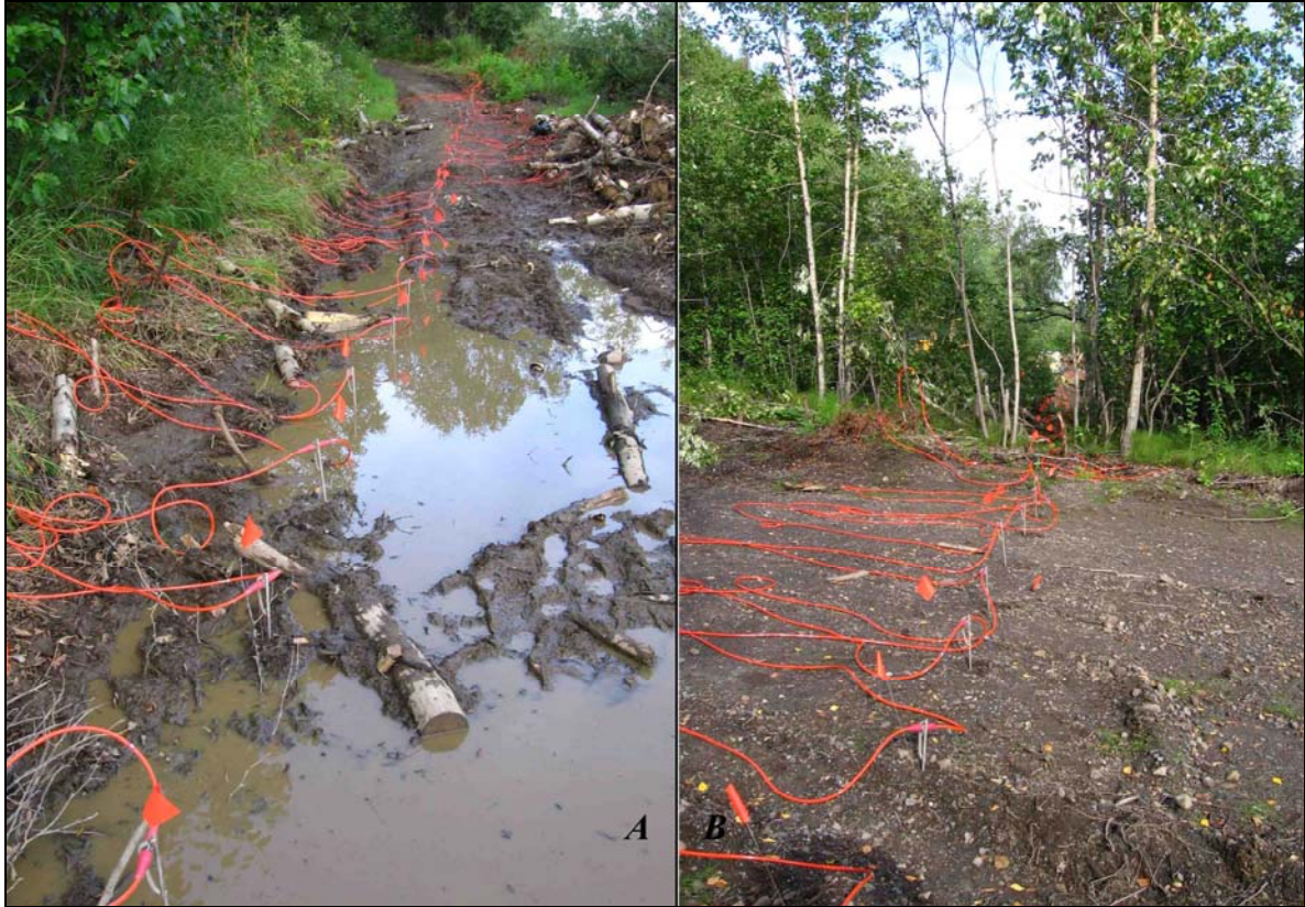
Figure 20. Photographs of the DC resistivity equipment deployed on line 7, (A) looking northwest along the access road and (B) from the southeast end of the line looking northwest toward Red Devil Creek in the trees.
